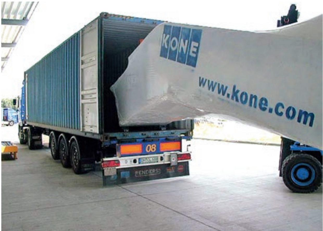
Figure 7.7 Unloading an escalator using forklift trucks
